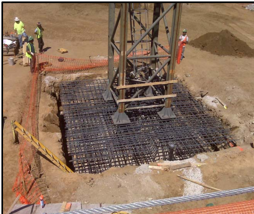
Figure 7: Crane Foundation Reinforcing, Barton Malow Site Photo
