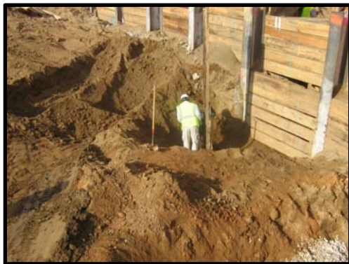
Figure 9: Sheathing and Shoring, Barton Malow Site Photo
